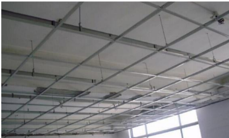
Steel frame on the ceiling
